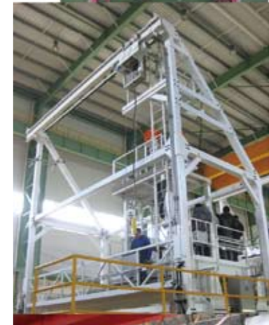
装卸料机 Fuel handling Machine
