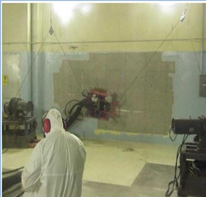
Figure 5. En-vac removing paint from wall in the Decon Shop
