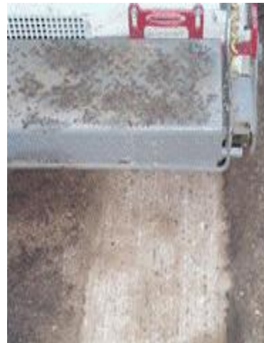
Milling cutter Allows single pass for thick ( several cm ) layer removal
