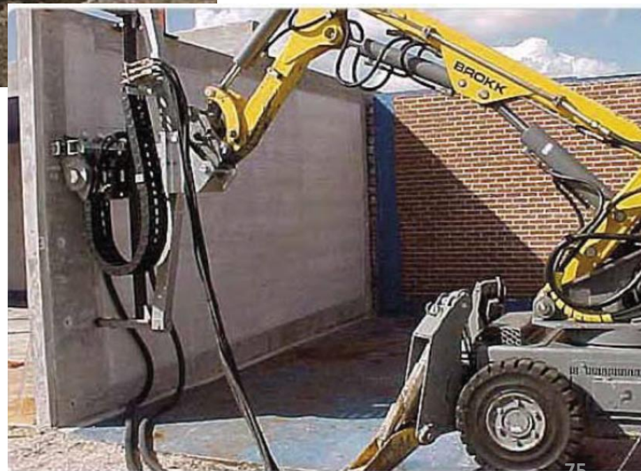
Floor Shaver(刨削機) mounted on Brokk 250 for 牆面去污
